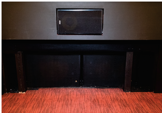
ADAMSON POINT 8 FRONT FILL ATOP TWO IS119 SUBWOOFERS BUILT INTO STAGE
