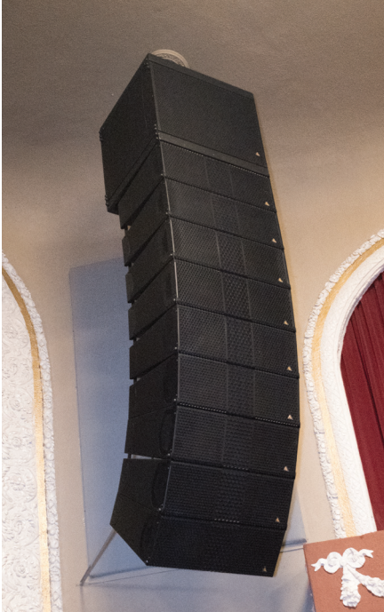
MAIN ARRAY OF NINE ADAMSON IS105 BELOW ONE IS119 SUBWOOFER
